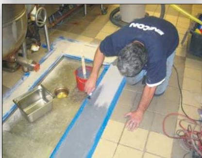
After damaged materials were removed, DuraQuartz was applied to provide a smooth transition from the quarry tile floor to the rim of the trough.
