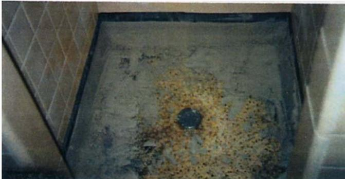
*Leaking existing terrazzo shower pan. Note tape applied above the first course of tiles to neatly define the DuraQuartz repair.*
