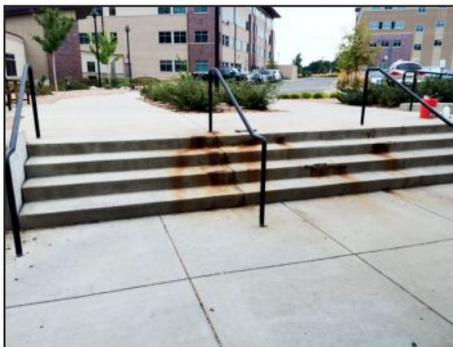
After only 12 years in use this staircase was cracked, crumbling and badly stained from the harsh elements and routine de-icing efforts during the harsh Colorado winters.
