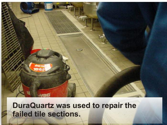
DuraQuartz was used to repair the failed tile sections.
