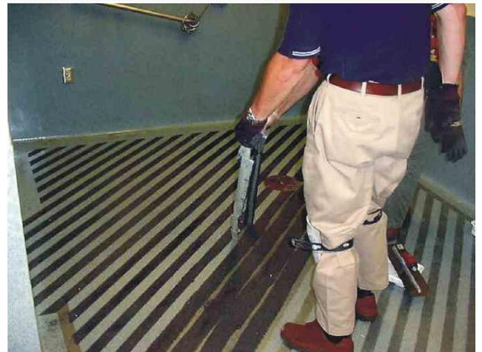
**CHEMCLAD SC + fine aluminum oxide [Al<sub>2</sub>O<sub>3</sub>] aggregate was used to provide slip protection for patients as well as therapists. This entire project was completed in just one day.**
