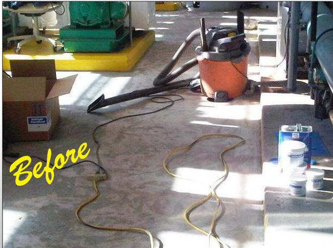
**Problem:** The original coating on this 2900 sq. ft. mechanical room floor was flaking and chipping. The concrete had also begun to crack and spall in several areas.
